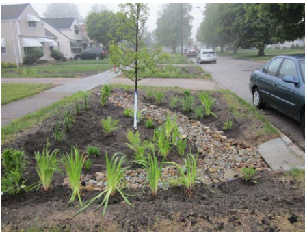
Klusner during construction
