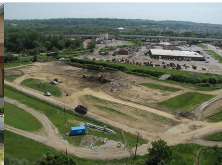
Confluence Project during construction
